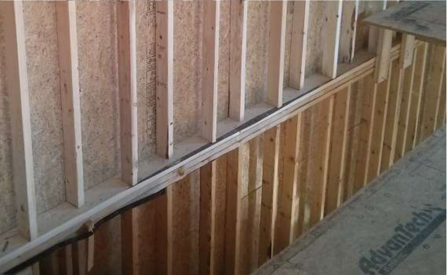
TYPICAL EXTERIOR FRAME WALL CONSTRUCTION
